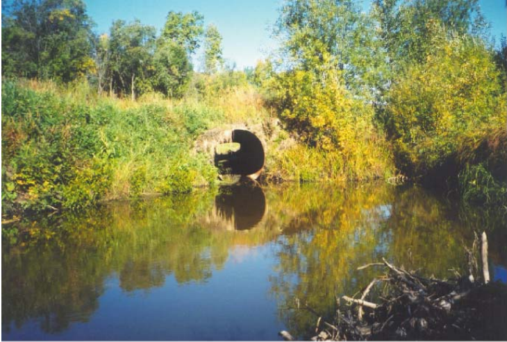
Plate 45. View of culvert outlet downstream of road (September 17/2002).
