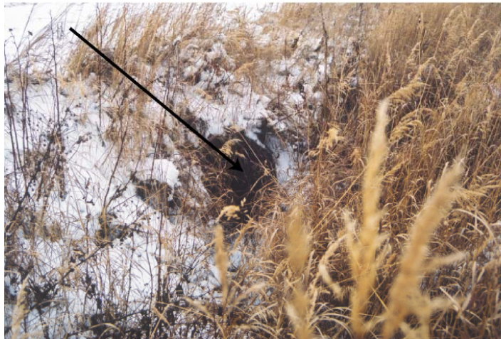
Plate 89. Upslope end of culvert. This culvert is mainly draining the ditchline. The ditchline is fairly well grassed; thus, crossing is probably contributing little if any to sediment load (November 12/2002).
