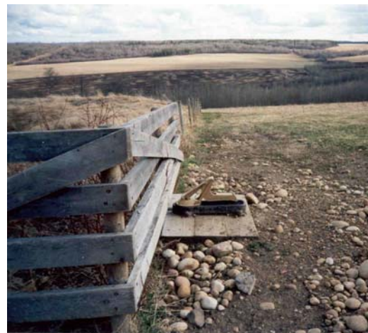
Aquamat pump installed at Glenn Hogbergs
