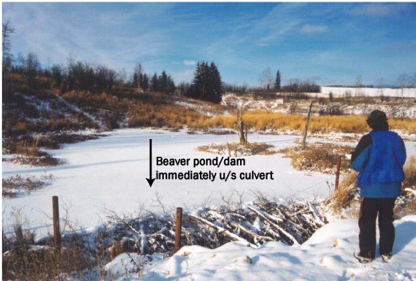
Plate 7. Series of beaver ponds upstream of road. Note beaver dam in forefront of photo (built in the culvert inlet). The ponds are extensive and if breached could result in torrential downstream flows and erosion (November 11/2002).
