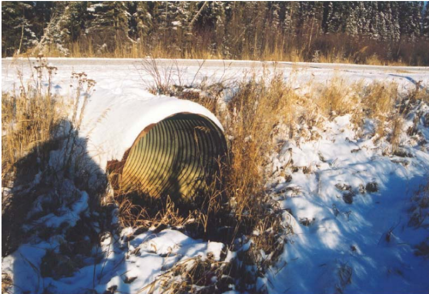
Plate 33. View of culvert upstream of road (November 11/2002).
