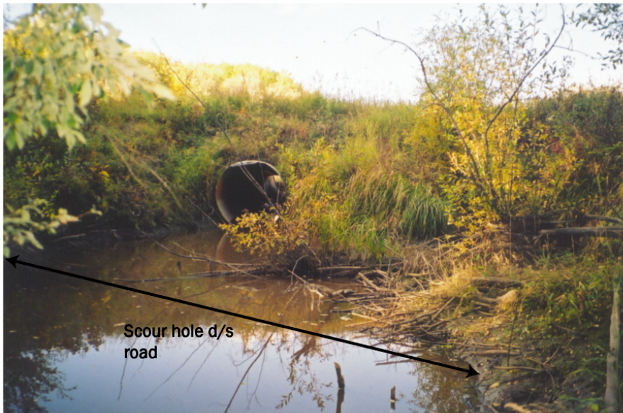
Plate 41. View of culvert downstream of road. Note highly turbid water (evidence of sediment transport) (September 16/2002).
