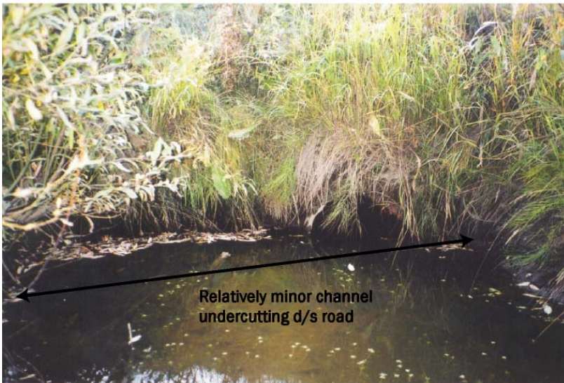
Plate 76. View of culvert outlet downstream of road. Note that there is some channel undercutting, but that riparian grasses and shrubs are providing some resistance to erosion. Bottom of culvert is flush to bottom of channel, i.e., not perched (September 19/2002).
