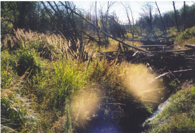
Plate 54. Channel immediately downstream of road is protected from erosion by a dense mixture of grasses, shrubs and dead woody debris (September 17/2002).
