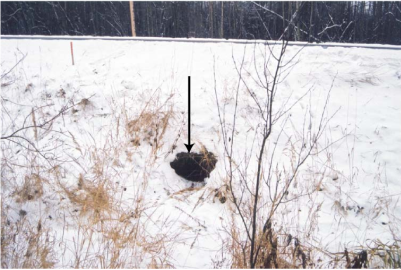
Plate 95. Culvert inlet upstream of road (November 12/2002).
