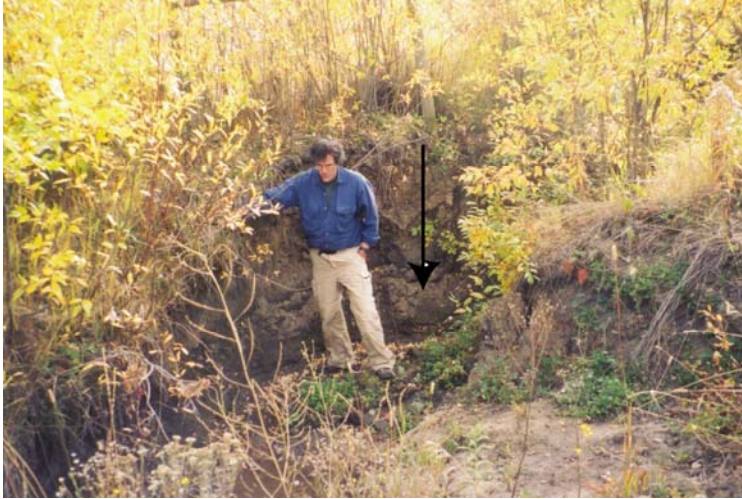
Plate 14. Sediment erosion down-slope of wellhead drainage pipe continues for considerable distance.
