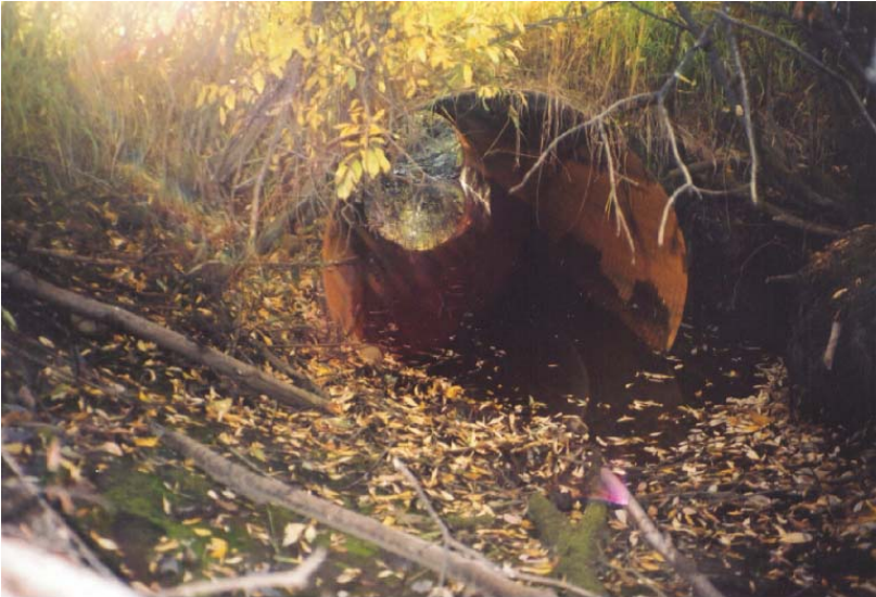
Plate 24. View of culvert outlet downstream of road. Note that the culvert outlet is compressed to channel bottom, i.e., it is not perched (September 17/2002).
