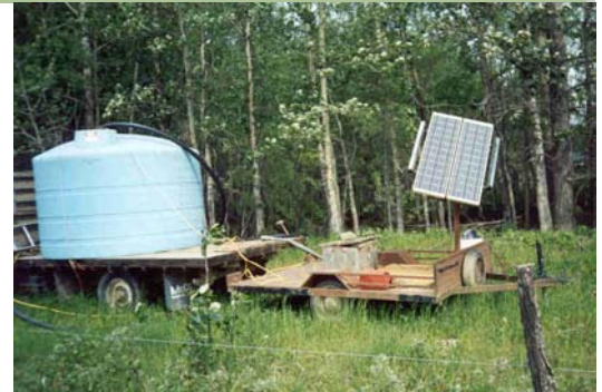
Solar system setup at Fred Burres
