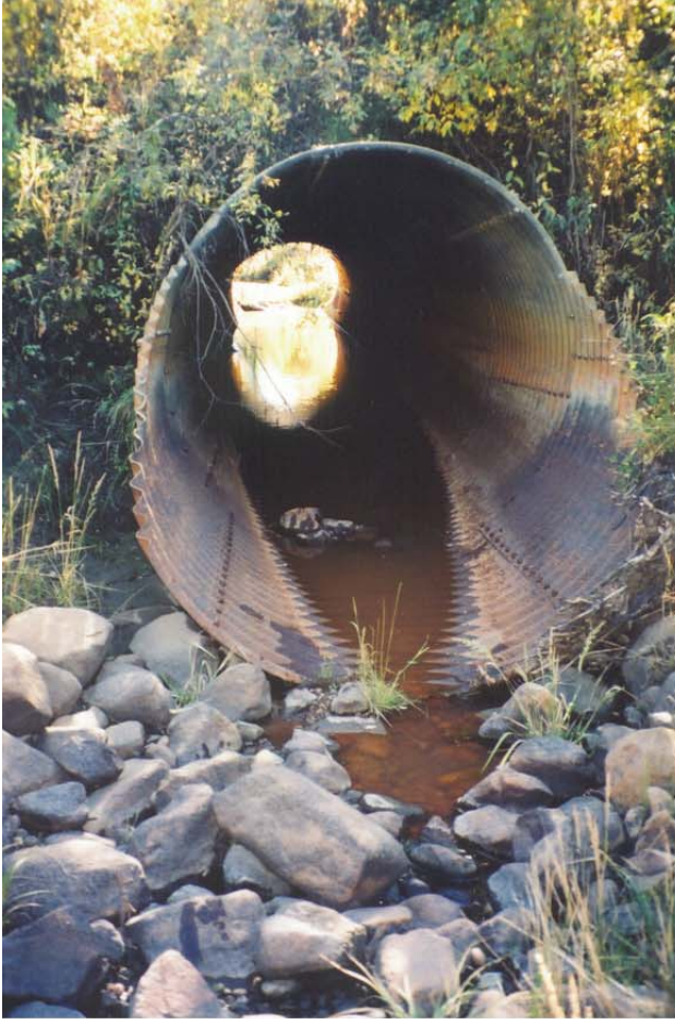
Plate 53. Inlet of culvert upstream of road. Note that bottom of culvert is flush with the bottom of the channel (not perched) and that large rocks have been used to stabilise soils at the road (September 17/2002).
