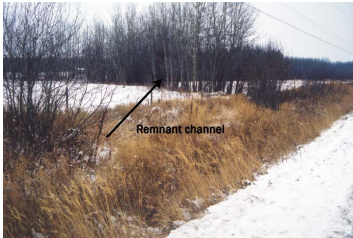
Plate 88. Upstream view of channel. At present, the culvert is draining primarily the ditchline; however, there may be a remnant channel running parallel to treeline in background (November 12/2002).
