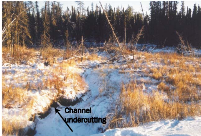
Plate 2. Channel undercutting downstream of road. Note that riparian grasses and shrubs are not of sufficient density to provide much in the way of channel protection (November 11/2002).
