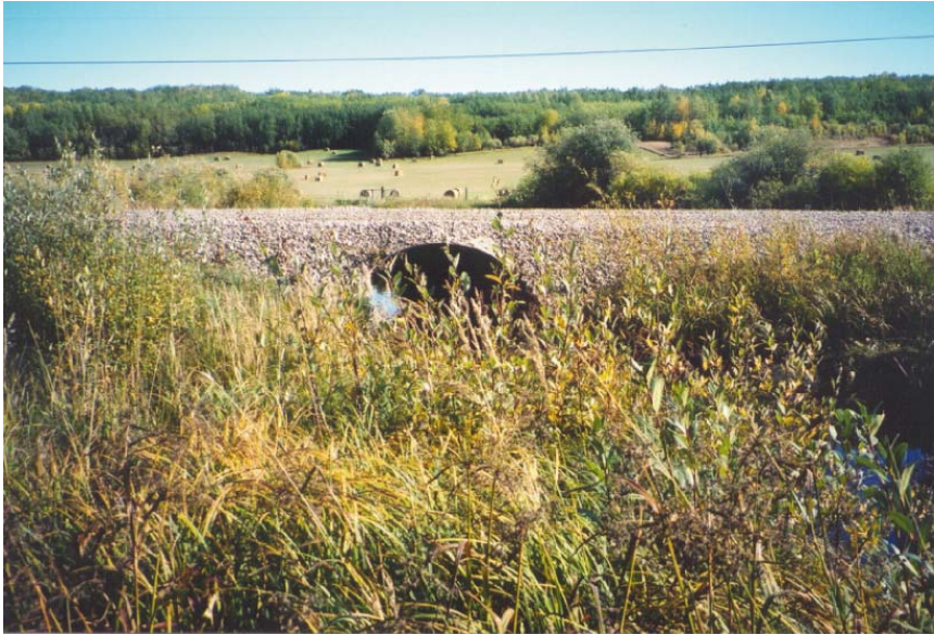
Plate 57. Culvert downstream of road showing upstream fields and riparian shrubs (September 17/2002).
