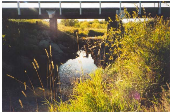
Plate 21. View downstream of road looking upstream (September 17/2002).
