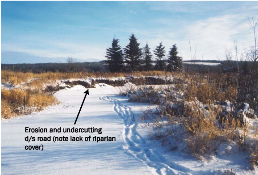
Plate 6. View of channel approximately 50 m downstream of road. Note that there is evidence of severe slumping on outside bend of the channel (riparian grasses are not sufficient to protect channel from erosion) (November 11/2002).
