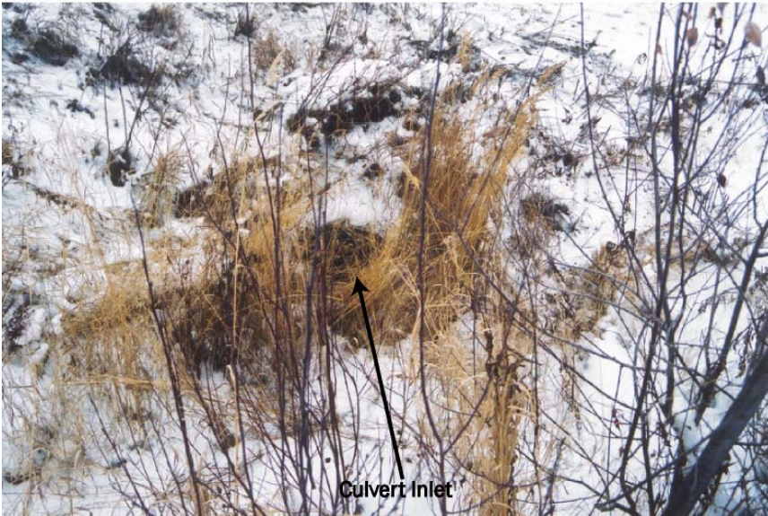
Plate 36. View of culvert inlet immediately upstream of road (November 12/2002).
