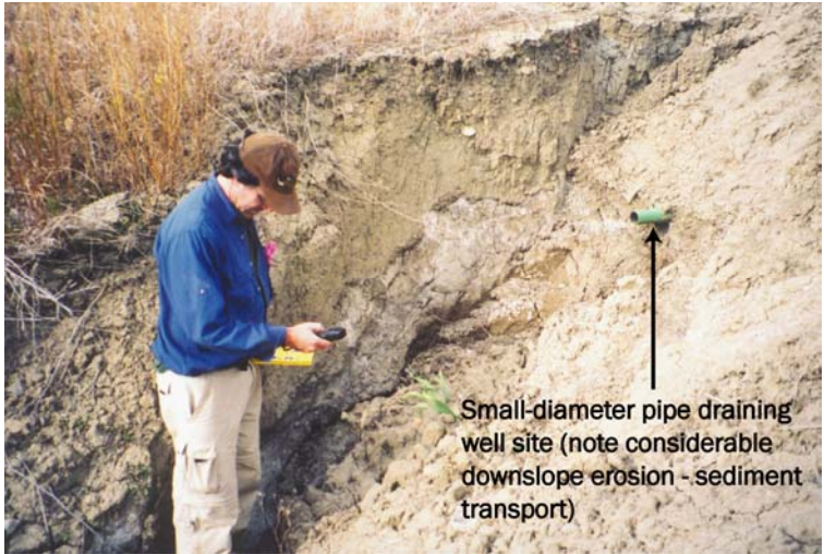
Plate 13. Small-diameter pipe that drains retention ditch on down-slope perimeter of oil and oil and gas wellhead. Note extensive sediment erosion resulting from the force of water through pipe.
