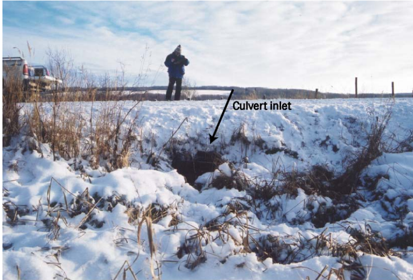
Plate 10. Culvert inlet upstream of road (November 11/2002).
