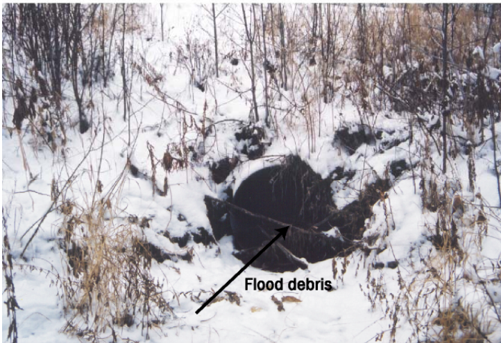
Plate 92. View of culvert inlet upstream of road. Note the flood debris hanging off the woody debris that is crossing the culvert and slumping behind the culvert (November 12/2002).
