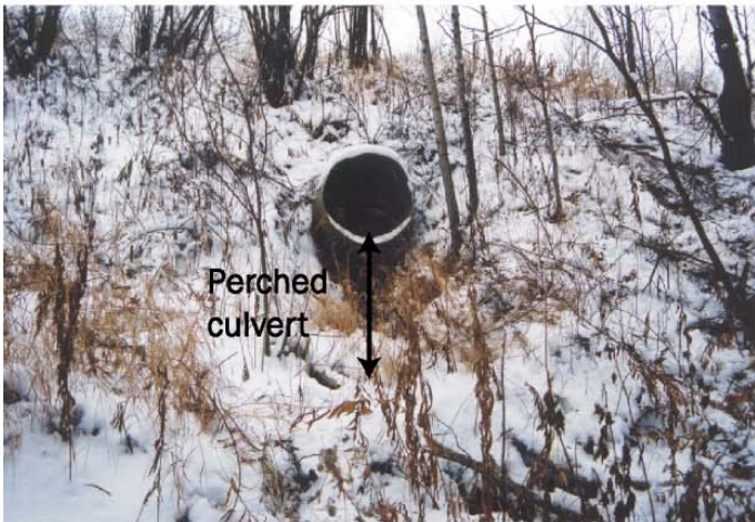
Plate 70. View of culvert downstream of road. Note that the culvert is perched (November 12/2002).
