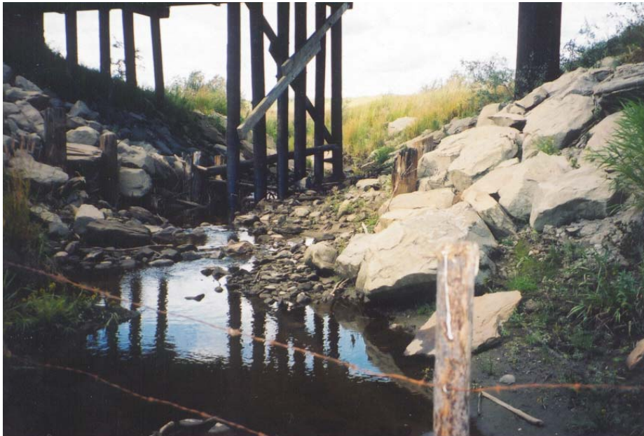
Plate 29. View downstream of bridge. Note the presence of large boulders used to protect channel from erosion (September 17/2002).
