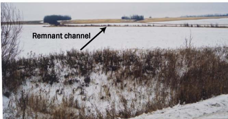
Plate 87. View upslope of road. At this time, the culvert probably just drains the ditchline (no apparent channel). The old channel can be seen in the far distance (November 12/2002).
