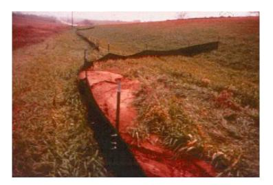
Figure 14 – Silt fence installed in a J-shape
