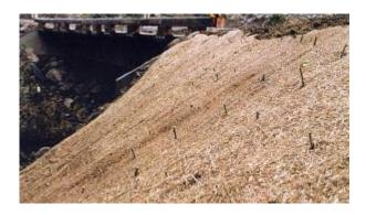
Figure 12 Installation of grass seed, coconut erosion control blanket and live willow stakes
