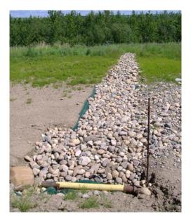
Figure 9 - Lining of drainage pathway from dyke drain
