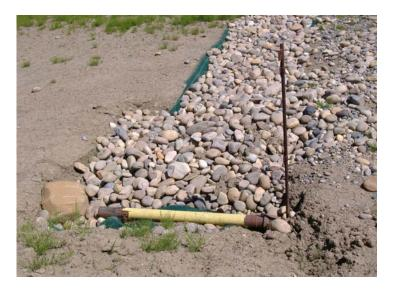
Figure 4 – Drainage pathway reinforced by geotextile and rip-rap
