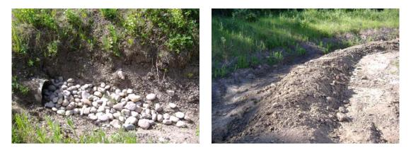
Figure 3 – Culvert rip-rap and berm repairs to control water
